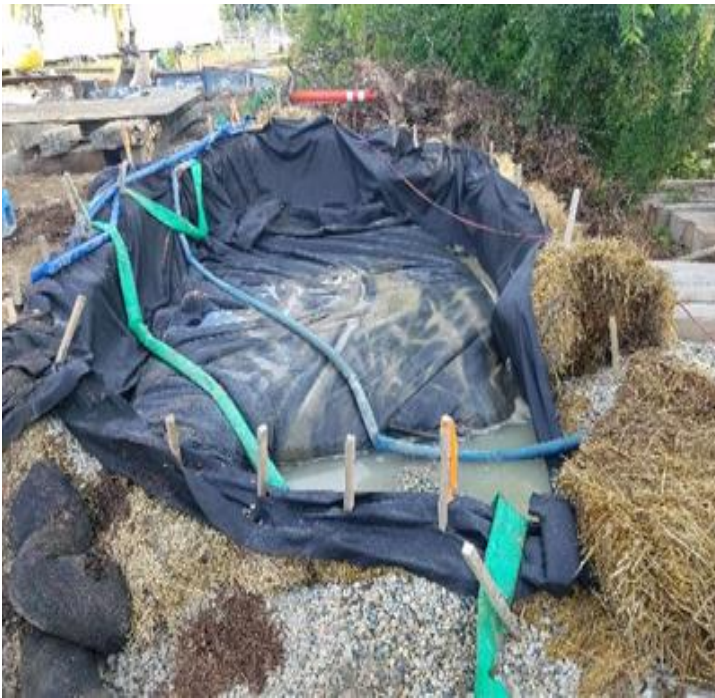
Fig 7: Geotextile filter fabric installed in dewatering apparatus. Viewing north. (8-12-19).
