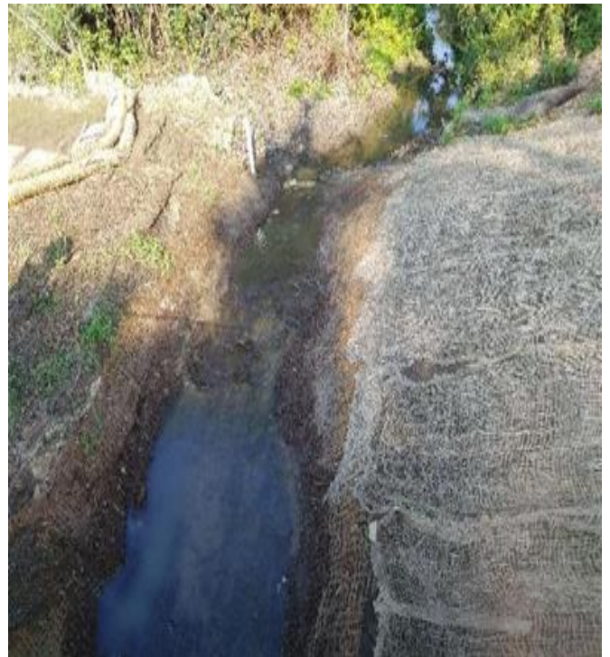
Fig 12: Repairs made to jute liner / blanket in College Brook. Viewing west. (8-13-19).
