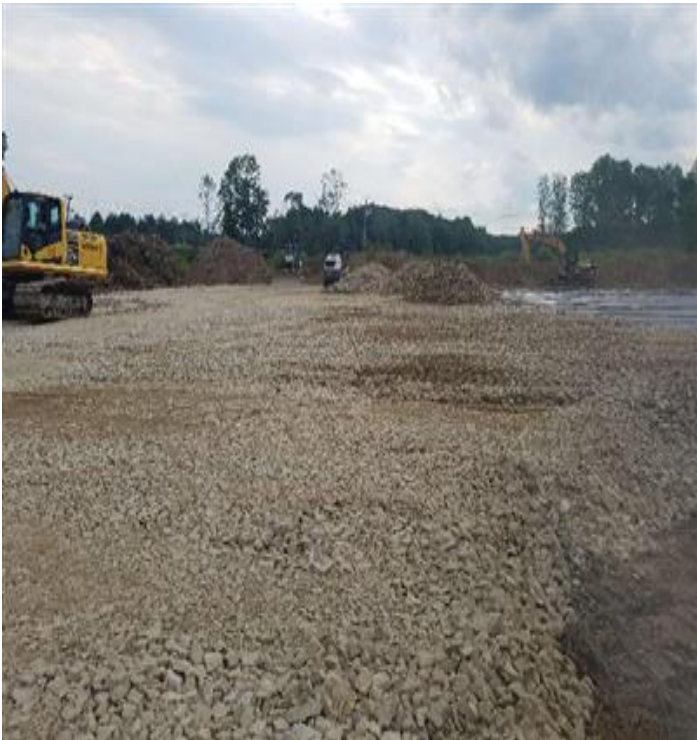
Fig 15: Progress of the Shattuck Road laydown area. Viewing west. (8-13-19).
