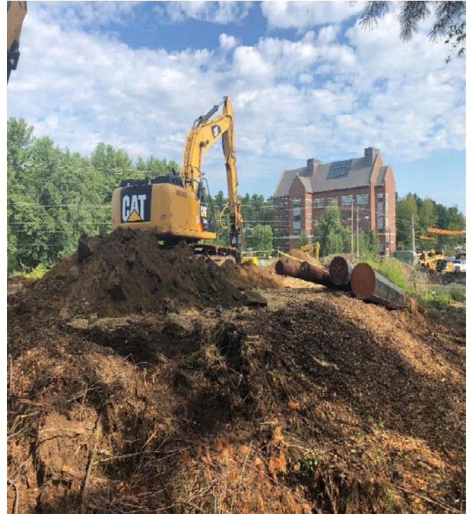
Fig 18: Excavating for Str. 25. Viewing north. (8-14-19).
