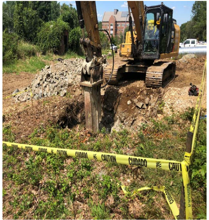
Fig 6: Began excavation for Str. 26. Viewing north. (8-10-19).
