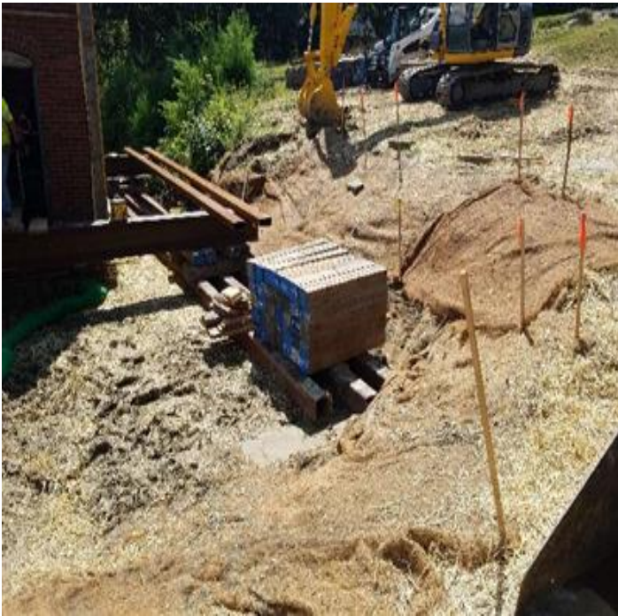
Fig 1: Maintaining blankets around cable house. Viewing south. (8-09-19).
