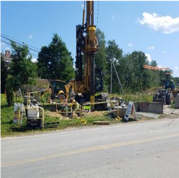
Fig 3: Drilling Str. 24. Viewing southeast. (8-09-19)
