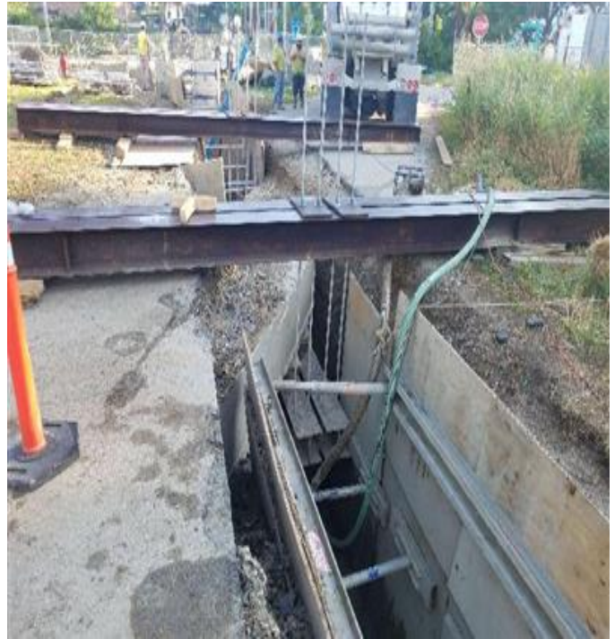
Fig 10: Support beam for duct bank and trenching activities. Viewing north. (8-12-19).
