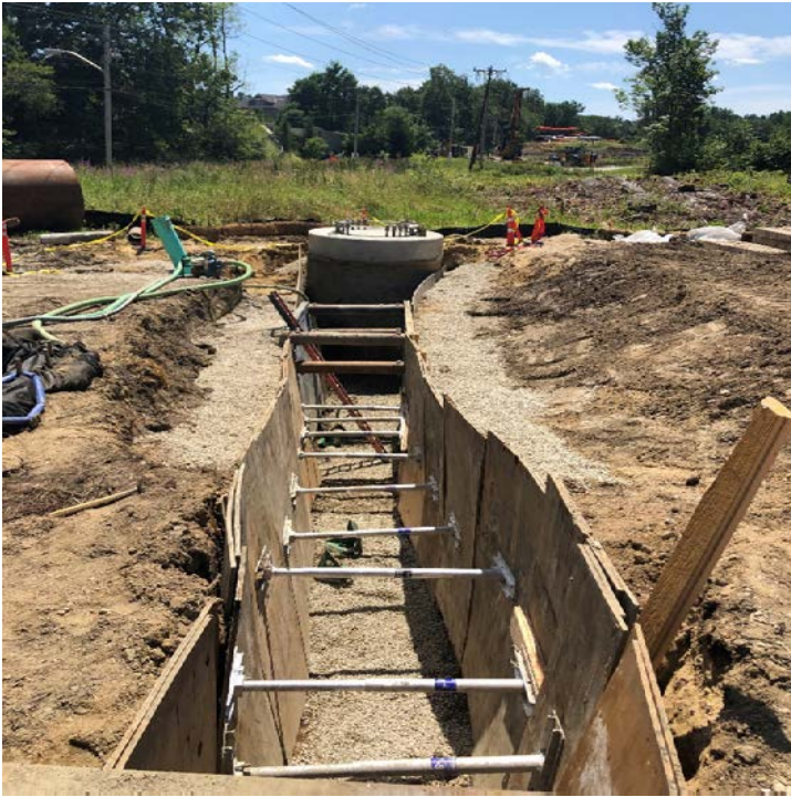
Fig 5: Trenching towards Str. 23. Viewing south. (8-10-19).
