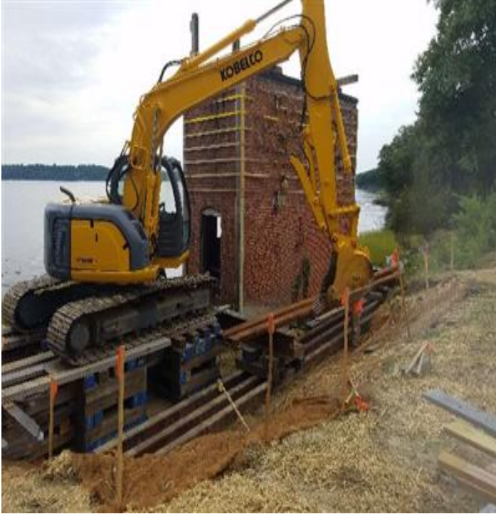
Fig 13: Gratan continues to assemble braces for the cable house. Viewing west. (8-13-19).
