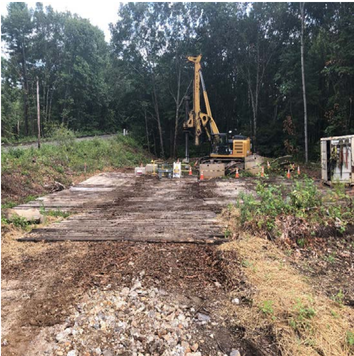
Fig 19: Prepping to drill Str. 30. Viewing south. (8-14-19).
