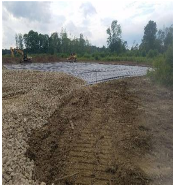
Fig 14: Progress of the Shattuck Road laydown area. Viewing west. (8-13-19).
