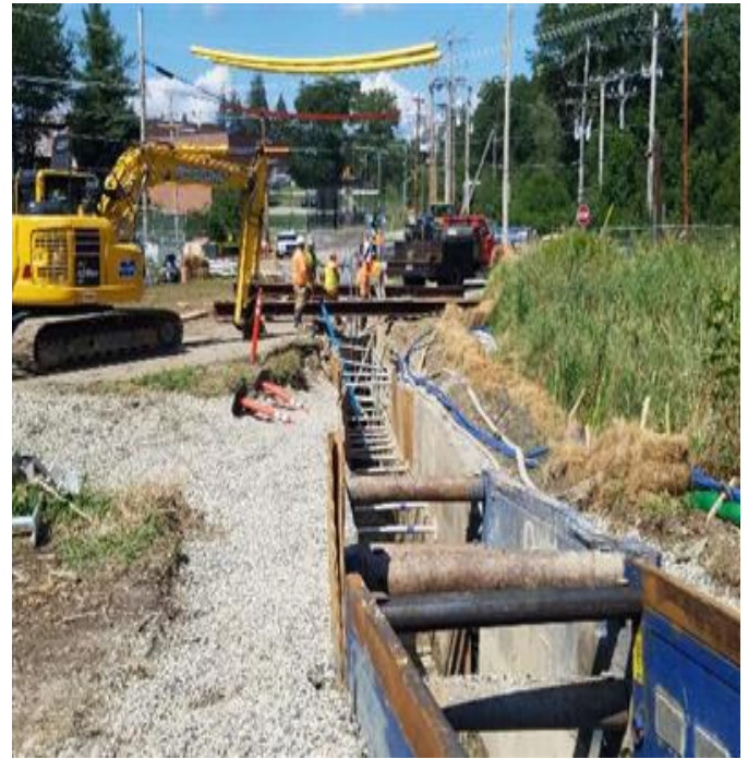
Fig 2: Trenching towards Str. 23. Viewing north. (8.09-19).
