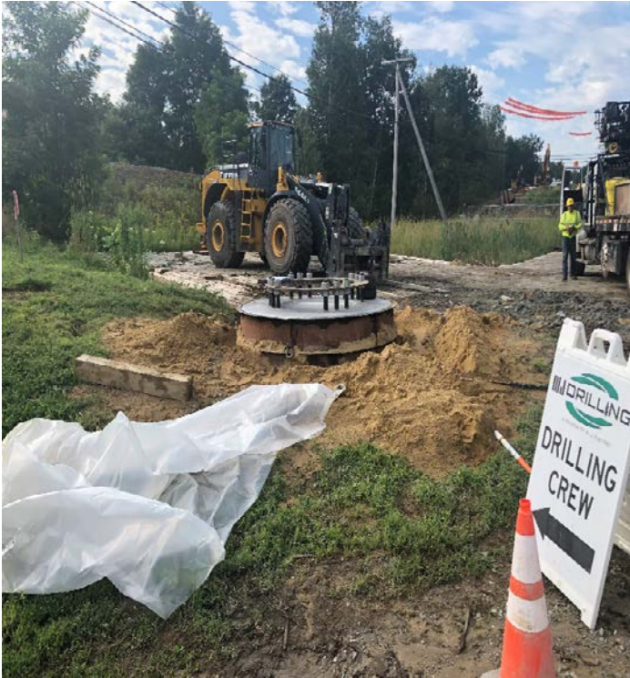
Fig 17: Str. 24 foundation. Viewing south. (8-14-19).
