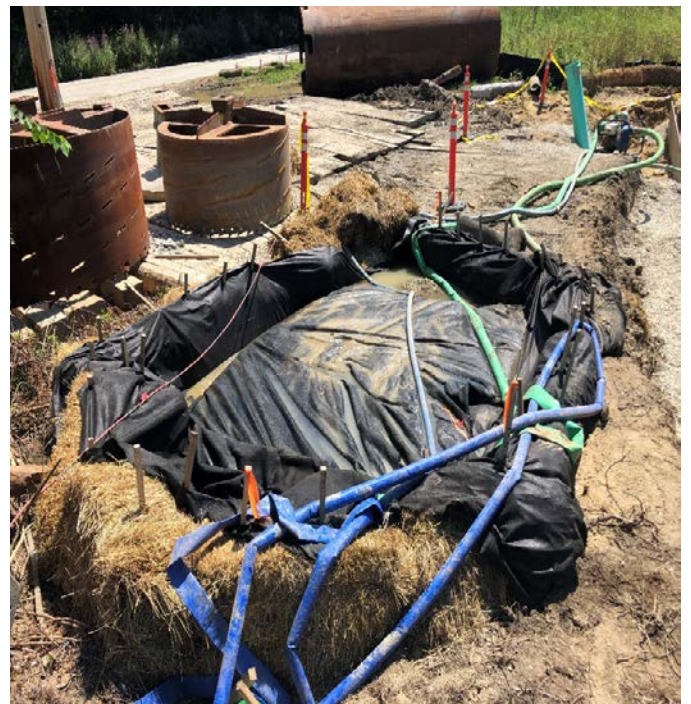
Fig 4 Geotextile fabric installed in dewatering apparatus at Str 23. Viewing south. (8-10-19).
